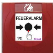
Smashing in the panel and pressing the button will only trigger an acoustic in-house fire alarm in order to alert other persons in the building to the situation. In addition to that, the fire department must be alerted via an emergency call by phone. The emergency call shall be made using the closest possible landline or a mobile phone. The emergency telephone number is 112.
